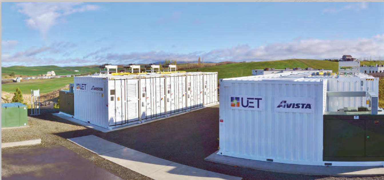
The 1 MW AC /4MWh AC Uni.System installed at Schweitzer Engineering Laboratories in Pullman, Washington
